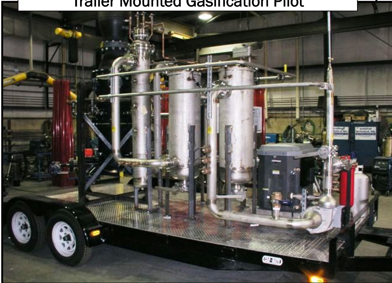
Trailer Mounted Gasification Pilot
