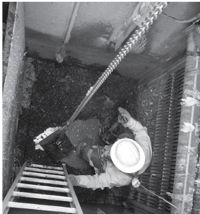
Confined space entry training makes this work a little easier.
