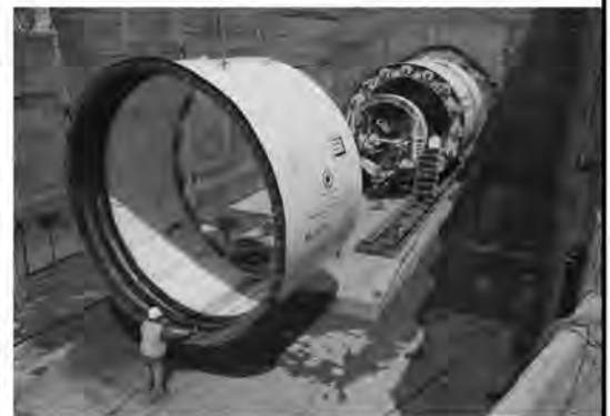
Henderson/ML King CSO Project and Pump Station, King County, WA
