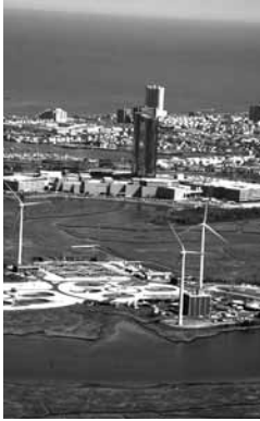
Wind turbine installation at the Atlantic County Utilities Authority (NJ) Wastewater Treatment Facility PHOTO CREDIT: MORTENSON CONSTRUCTION/LEE VERNON STUDIOS
