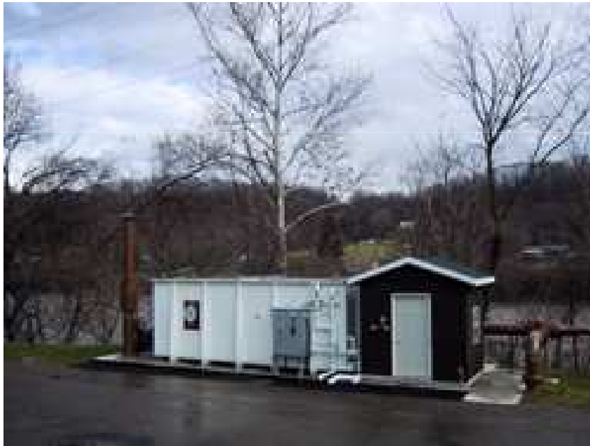
BASYS™ unit at Zanesville, Ohio
