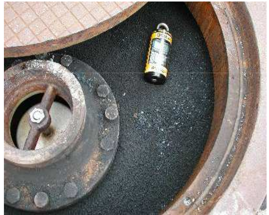
Force main air release manhole application in Johnson County, Kansas
