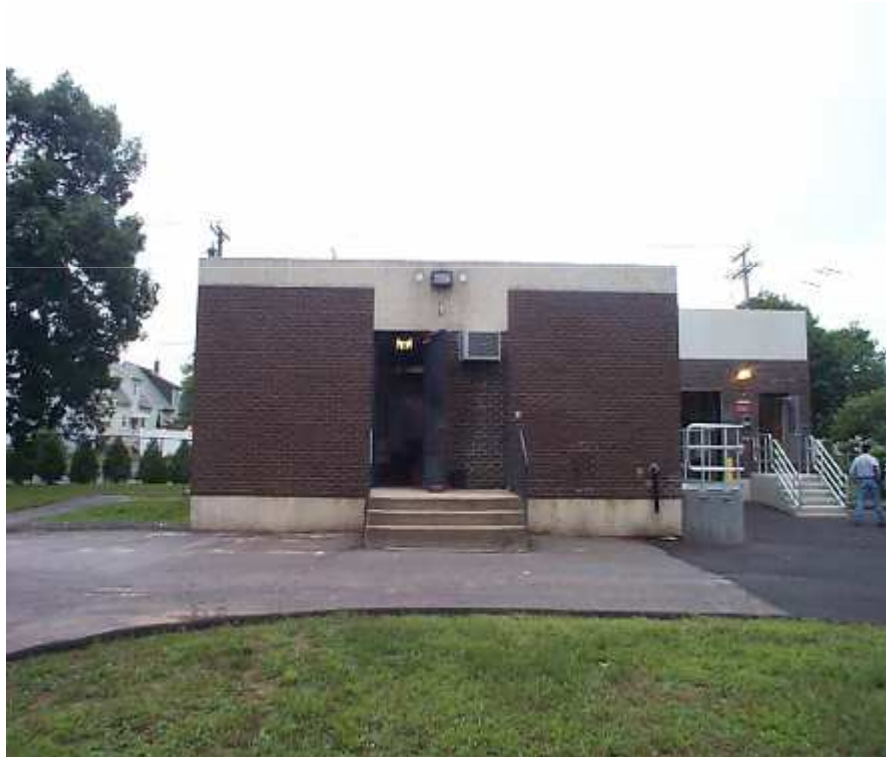
Westhaven Pump Station
