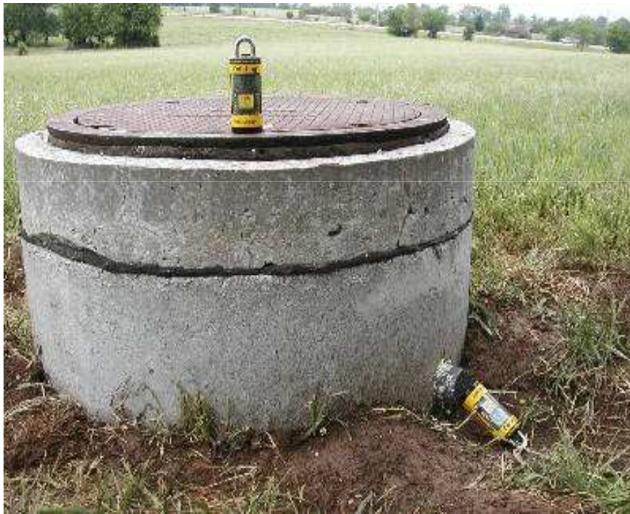
Force main air release manhole application in Johnson County, Kansas
