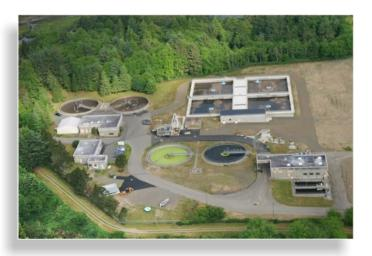
The plant now operates on a time mode system to try to maintain a constant effluent flow without pre or post equalization.
