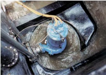
WEMCO-Hidrostal Prerotation System is a unique, economical, uncomplicated method of automatically adjusting pumping volume to varying inflow rates using a constant speed motor/pump.
