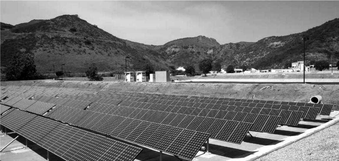
Solar Array at the Hill Canyon Wastewater Treatment Plant, Camarillo, California. The Array provides about 15% of the facility's energy needs.
